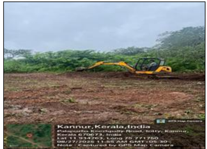
Fig 5: Area clearing for boundry fencing
